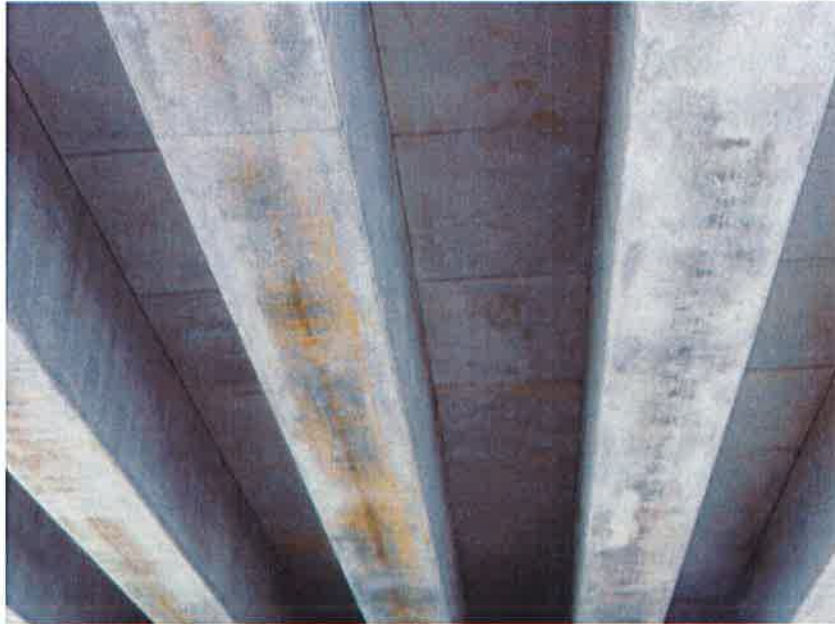
BOTTOM OF DECK
